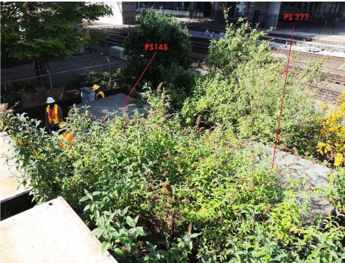
1b. Brush surrounding the switch adjacent to SW648 is so dense that it is not accessible.
