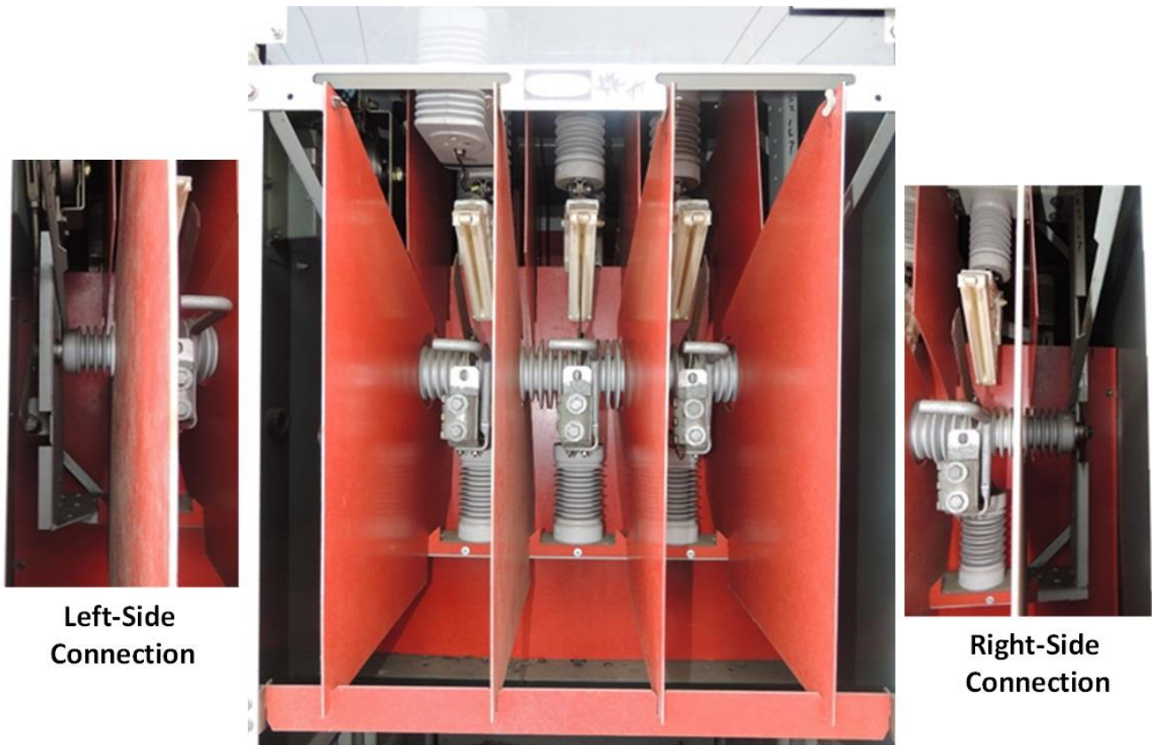
10b. Pre-2005 PMH Switch strut assembly. Note that the strut assembly runs the full length of the switch and is attached to the switch frame on both ends.
