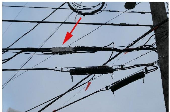
**Figure 4.9g. CATV line amplifier with coupler, WaveCom**
