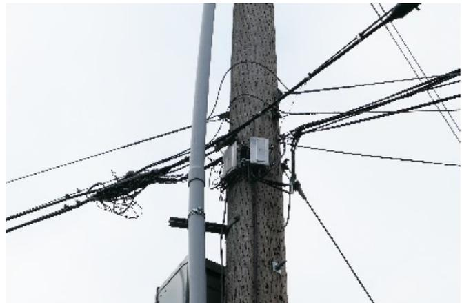
**Figure 4.8d. Serving terminal for telephone copper aerial cable, alternate style**
