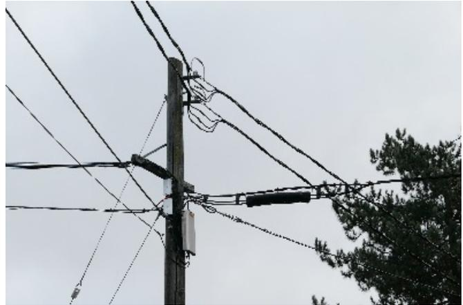
**Figure 4.8b. Serving terminal (silver box) and splice case (center right) for telephone copper aerial cable**
