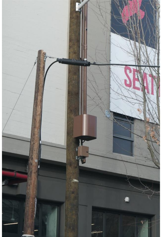
**Figure 4.1s. Power supply enclosure and service disconnect switch**
