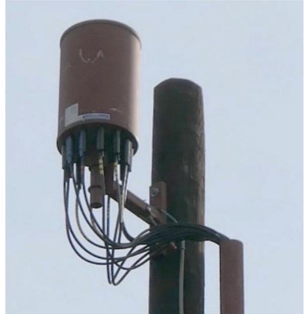
**Figure 4.1k. ★SWF antenna**
