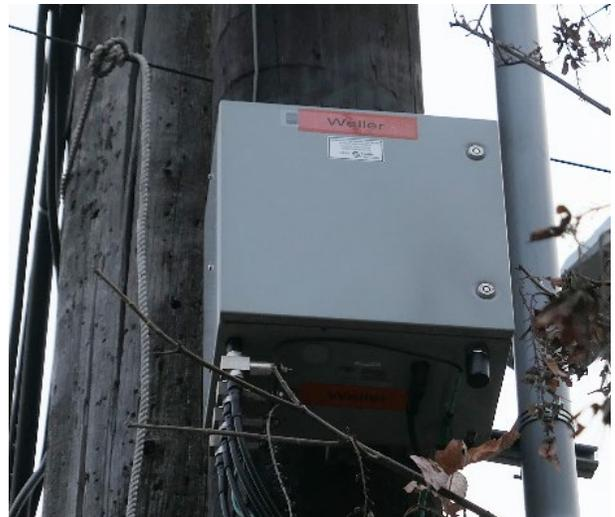
**Figure 4.7c. Communications enclosure for AMI collector**
