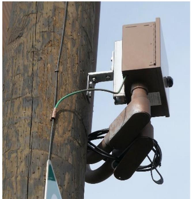
Figure 4.1f. Service disconnect switch enclosure for SWF, site still under construction
