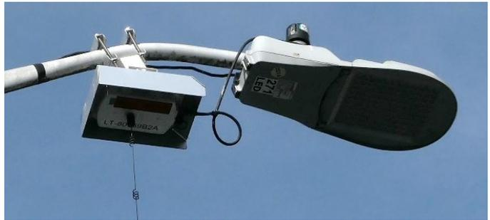
Figure 4.5b. ★ AMI repeater (router), SCL
