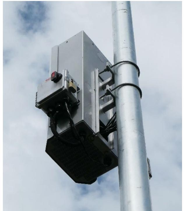
Figure 4.1v. SWF below streetlight bracket arm, co-located, enclosure
