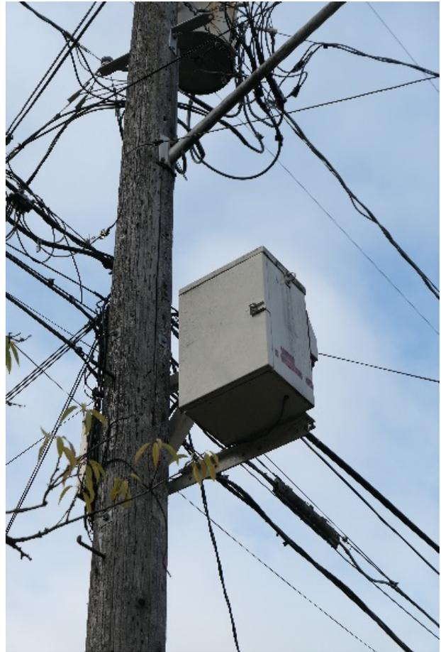
**Figure 4.1q. Power supply enclosure, no SWF on pole, location of service disconnect switch**
