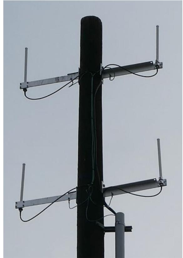
**Figure 4.7b. ★ AMI collector antenna, SCL**
