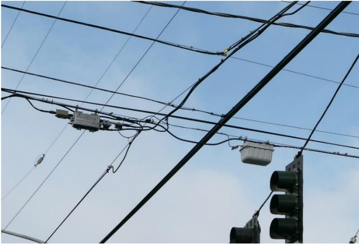
**Figure 4.3a. Strand-mount antenna, Wi-Fi hotspot (at right)**
