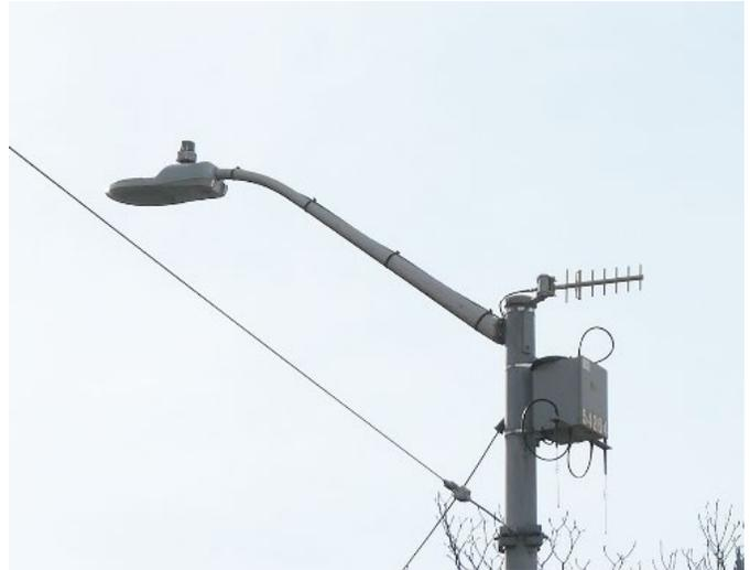
**Figure 4.6d. ★ AMR microcell controller with Yagi antenna, PSE**
