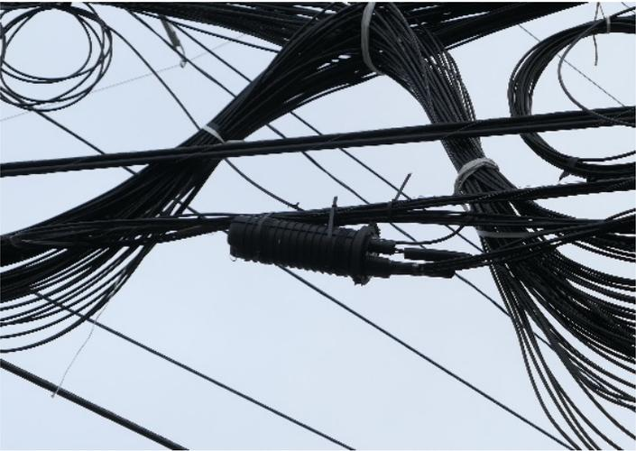
**Figure 4.8l. Fiber Optic Cable Splice**
