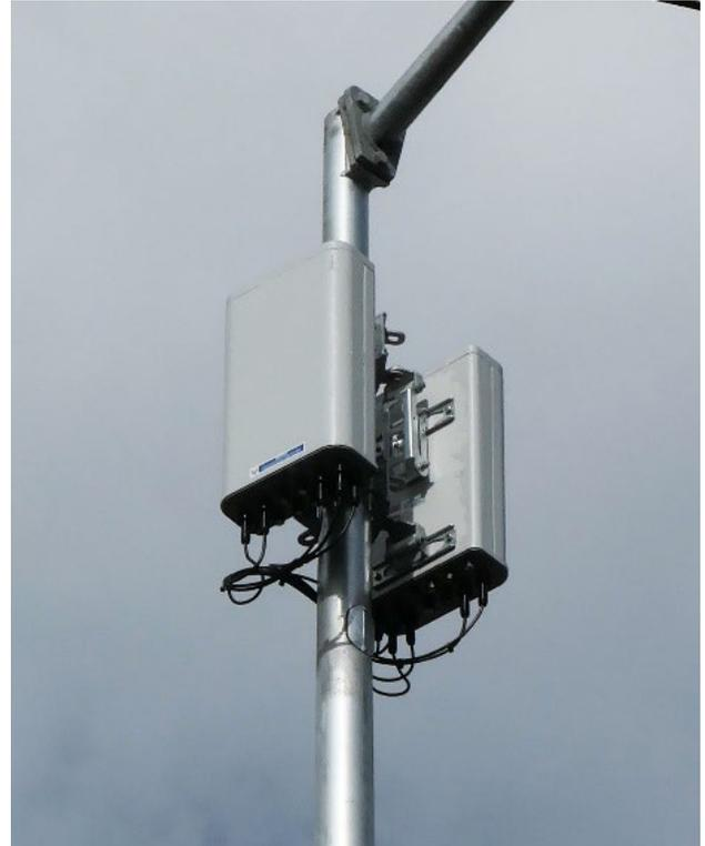
Figure 4.1u. ★ SWF below streetlight bracket arm, co-located, antenna
