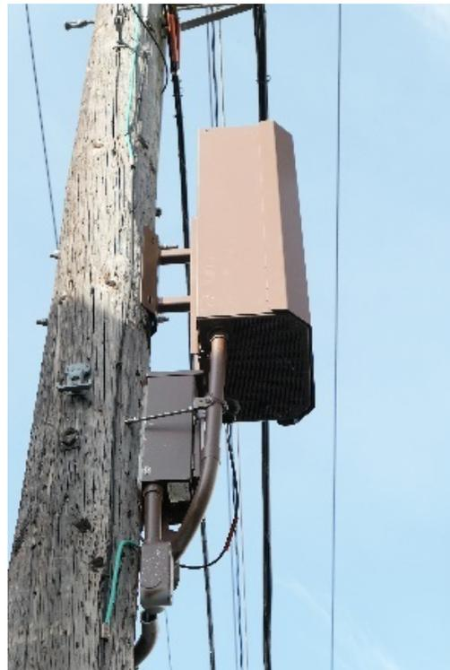
**Figure 4.1c. Power supply enclosure and service disconnect switch**
