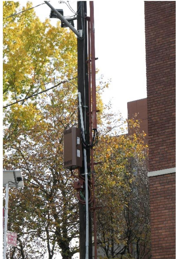
**Figure 4.1l. Power supply enclosure and service disconnect switch**
