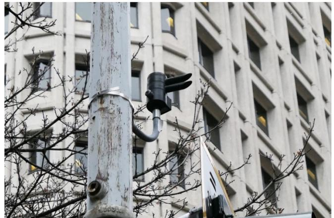
**Figure 4.12e. Traffic signal pre-emption sensor**
