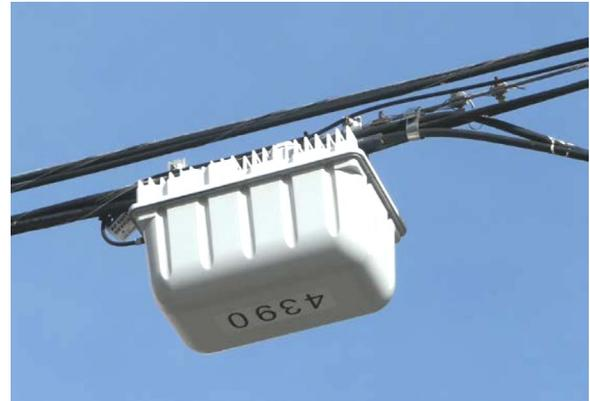
**Figure 4.3c. ★ Strand-mount antenna, Wi-Fi hotspot, Comcast, alternate view**
