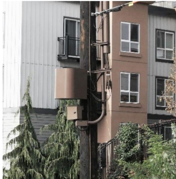
Figure 4.1i. Power supply enclosure and service disconnect switch
