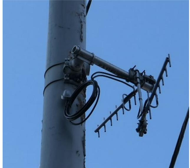
Figure 4.12i. ★ Yagi antenna for King County Metro Transit
