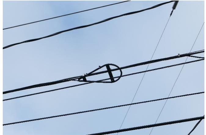
**Figure 4.8f. Fiber optic cable storage bracket
