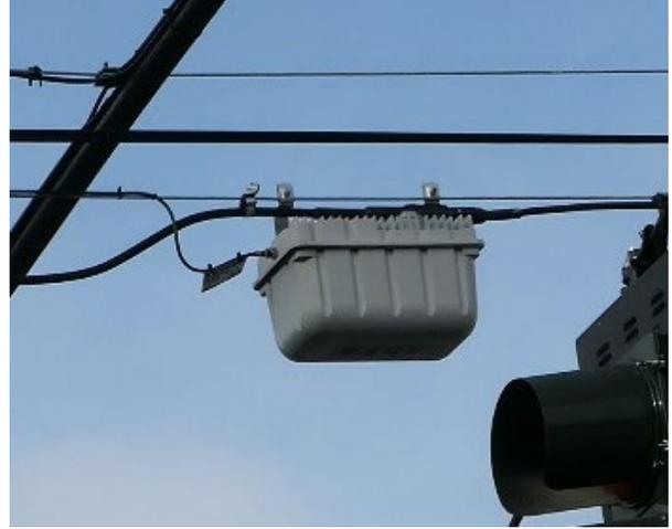
**Figure 4.3b. ★ Strand-mount antenna, Wi-Fi hotspot, Comcast**
