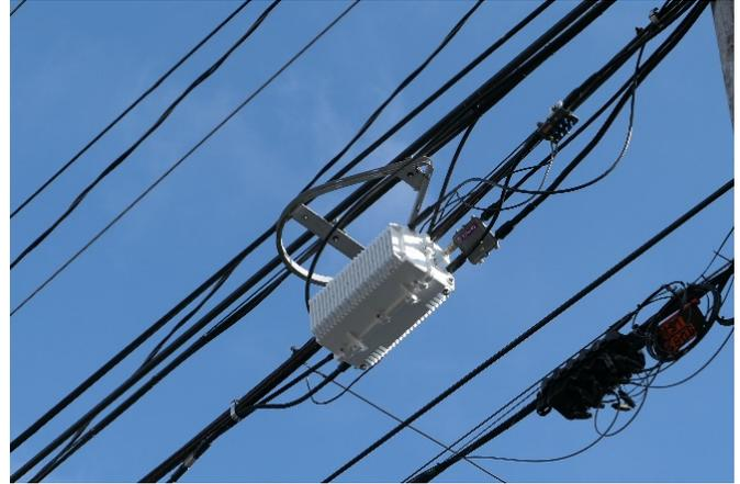
**Figure 4.9d. Node amplifier, Comcast**
