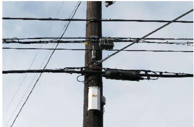
**Figure 4.8c. Serving terminal (silver box) and splice case (center right) for telephone copper aerial cable**
