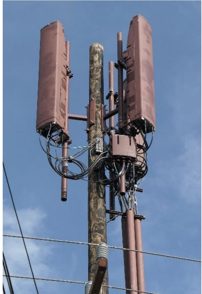
**Figure 4.4d. ★ Macrocell antenna, T-Mobile**
