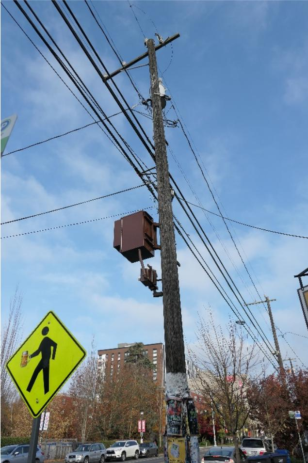
**Figure 4.1p. Power supply enclosure, no SWF on pole, location of service disconnect switch, Crown Castle**
