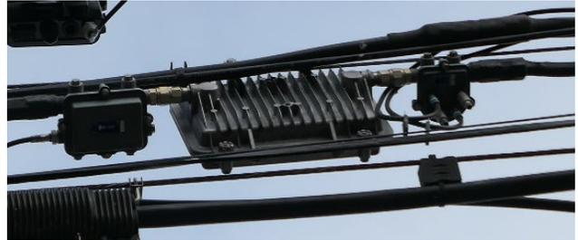
**Figure 4.9b. CATV line amplifier, with coupler, WaveCom**
