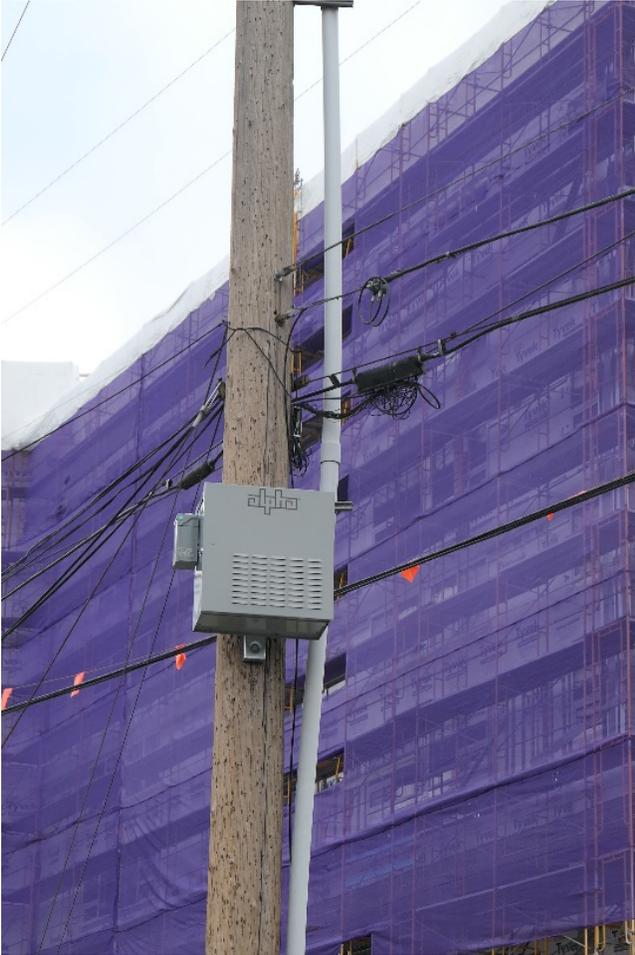
**Figure 4.1r. Power supply enclosure and service disconnect switch**
