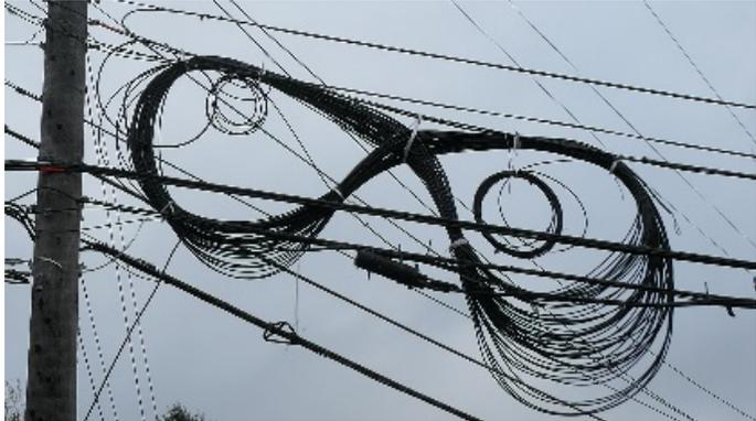
**Figure 4.8k. Fiber optic cable slack loop (aka Figure 8 storage) waiting to be put in halo**
