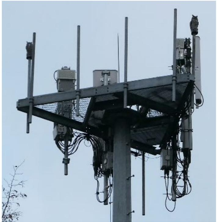
Figure 4.4b. ★ Macrocell antenna on non-SCL monopole
