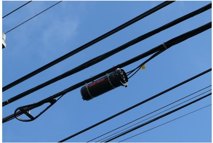
**Figure 4.8h. Fiber optic cable splice**
