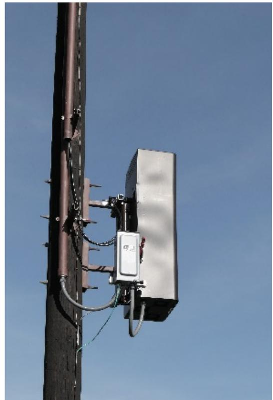
**Figure 4.1o. Power supply enclosure and service disconnect switch**
