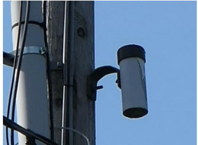
**Figure 4.12g. Spare low-voltage fuse storage container (obsolete), SCL**
