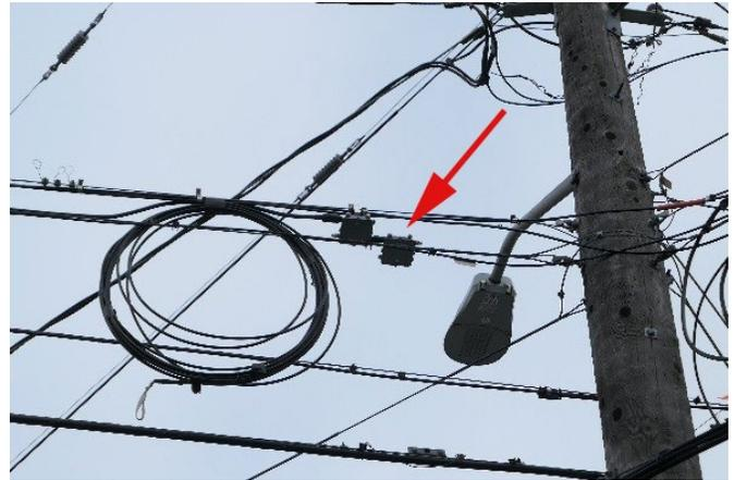
**Figure 4.9f. CATV cable coupler (non-active), Comcast**
