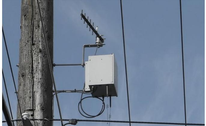
**Figure 4.6f. ★AMR microcell controller with Yagi antenna, PSE**
