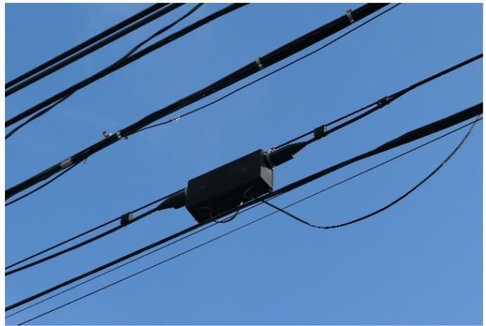
**Figure 4.8i. Serving terminal for telephone copper aerial cable**
