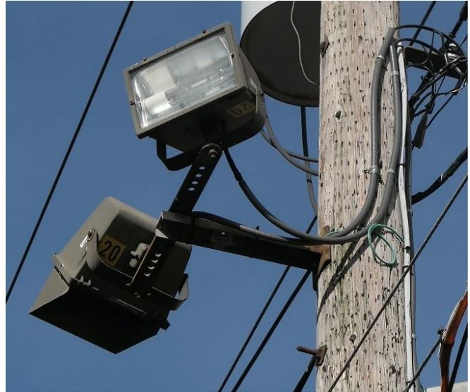
Figure 4.10b. Cluster-mount, high-pressure sodium (HPS) floodlights
