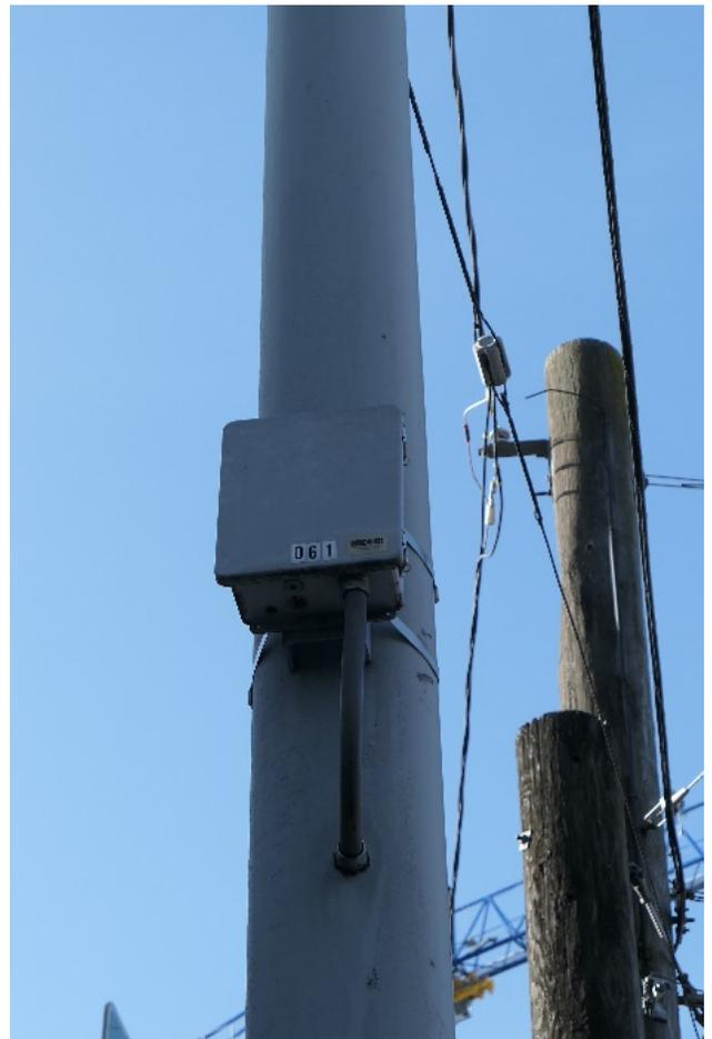
Figure 4.12j. Communications enclosure for King County Metro Transit Yagi antenna
