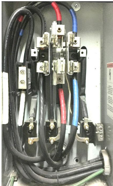
Figure 4. Proper Wire Configuration for Safety and Block Bypass Sockets
