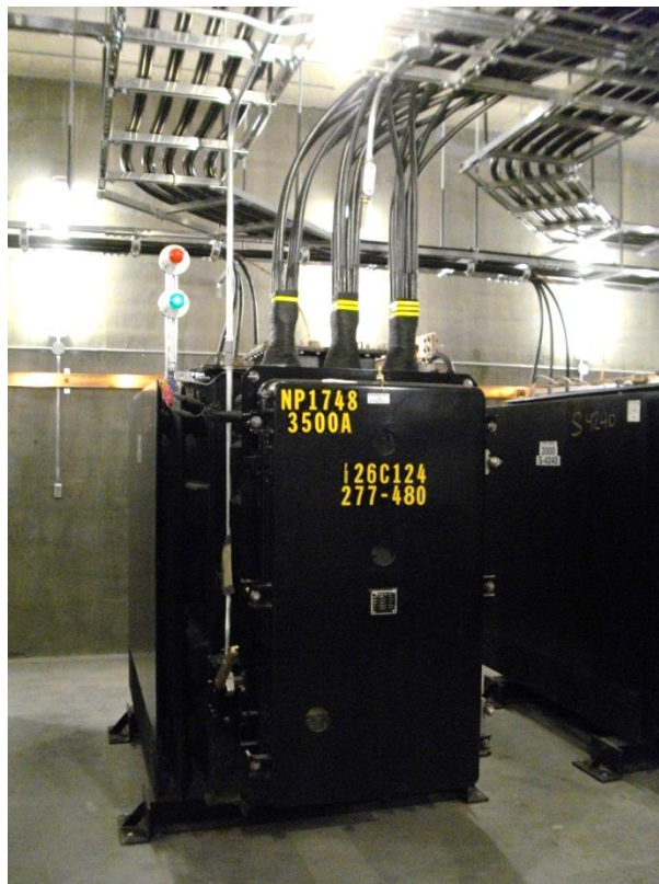
Figure 3.6a. Network Transformer
