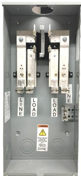
Figure 3c. Class 320 Block Bypass Socket
