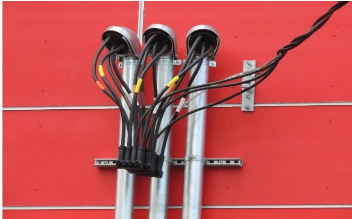
Figure 3.2b. Multi-Tap Insulated Connector, Stock. Nos. 013661 or 013662
