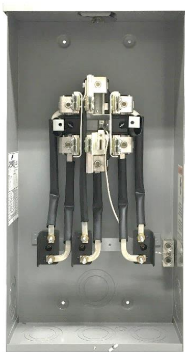
Figure 3c. Class 320 Block Bypass Socket
