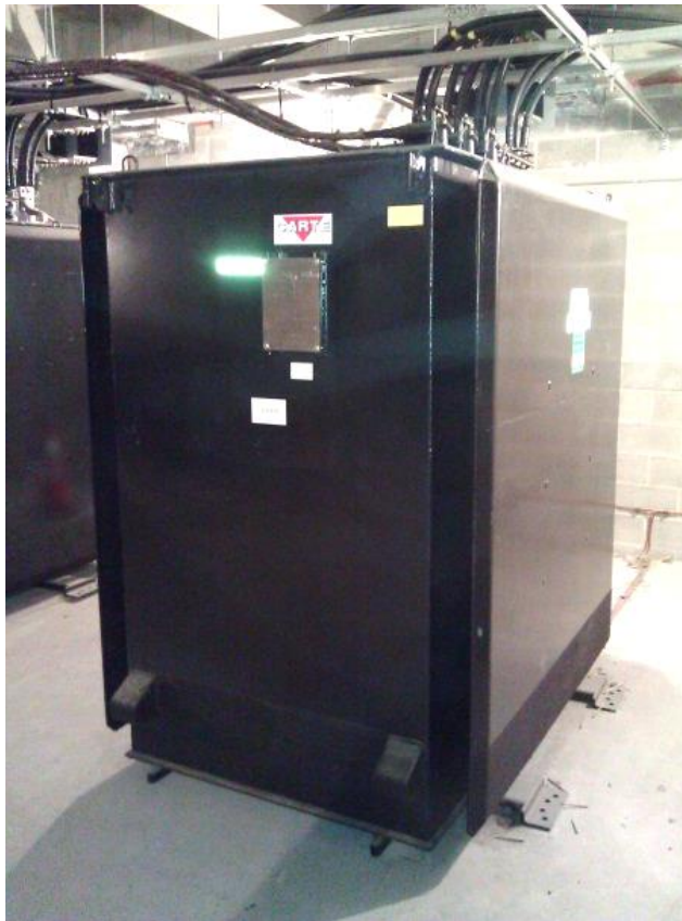
Figure 3.7a. Looped Radial Three-Phase Transformer
