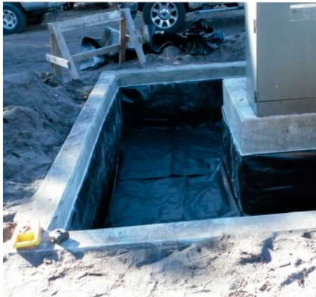
Figure 8b. Basic Concepts Geomembrane/Barrier Boom or SorbWeb Plus Blankets
