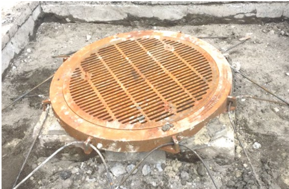
Figure 3a. Rebar Hairpin Example
