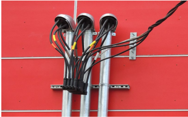
Figure 3.2b. Multi-Tap Insulated Connector, Stock. Nos. 013661 or 013662
