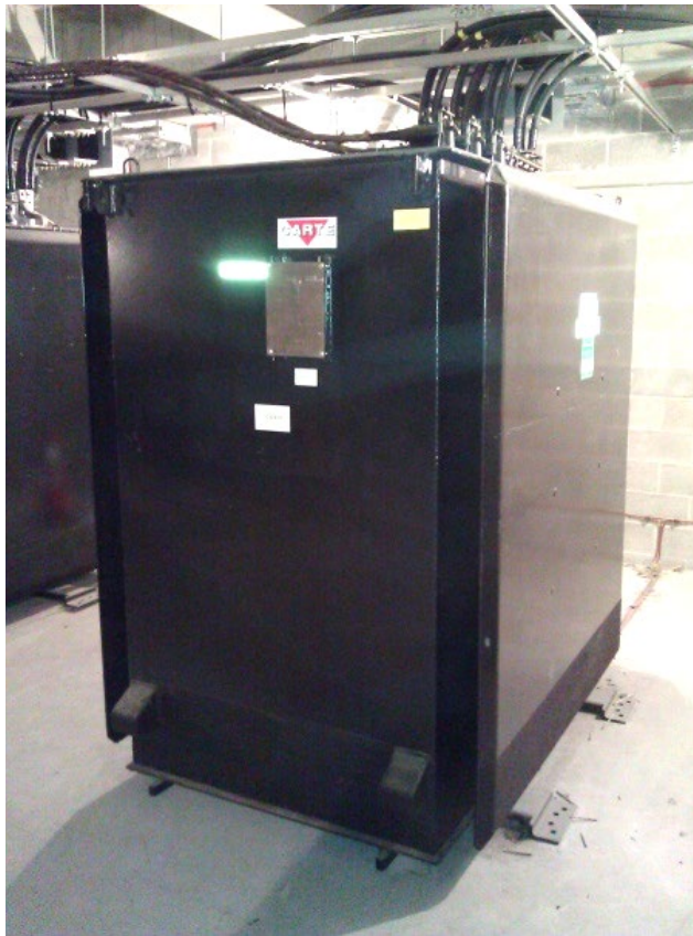
Figure 3.7a. Looped Radial Three-Phase Transformer
