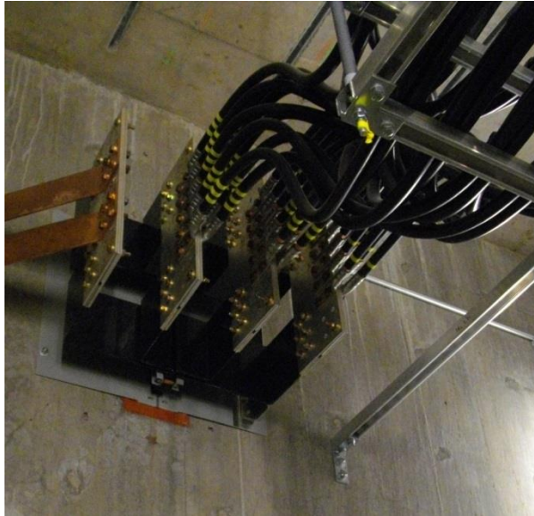
Figure 3.10e. Bus Bars Perpendicular to Floor, Plan View
