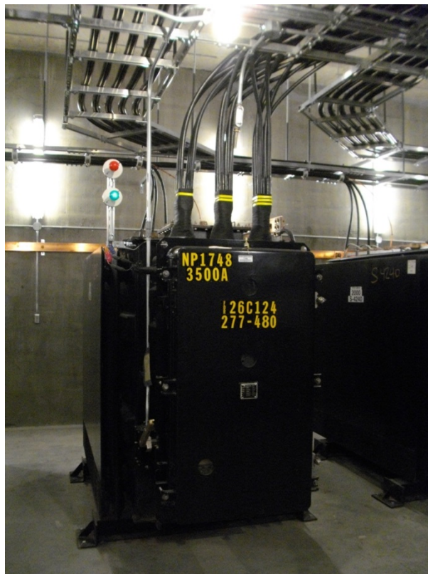
Figure 3.6a. Network Transformer
