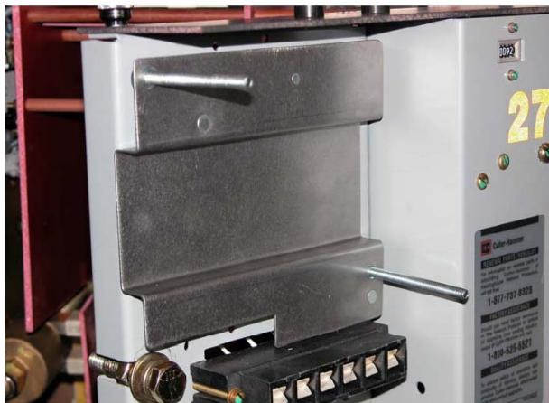
Photo W5 – NCS Transmitter Bracket Part No. DG-5003 in NWP
