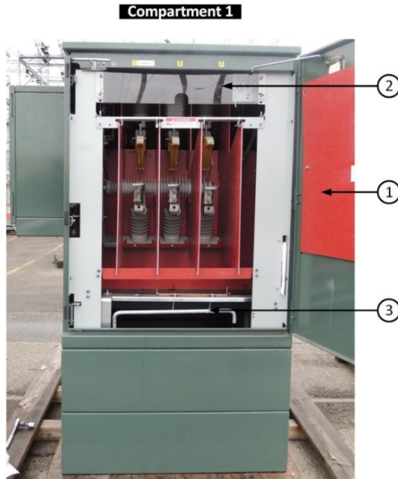
Figure 4b. PMH-5 Switchgear Compartment 1 Detailed View
