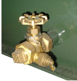
Figure 6.13.6. Drain Valve
