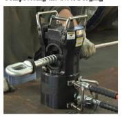
After the steel forging is compressed, care should be taken to secure the forging assembly to the rigging to not allow the conductor to be dropped. This can cause stress on the 3M ACCR core wires.
