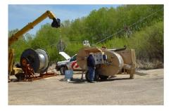
Never install 3M ACCR using a 'V-Groove' type tensioner. Use of V-Groove type tensioner may damage the inner core wires of the 3M ACCR.
