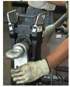
After the entire dead-end body is completely pressed on to the 3M ACCR, take care to secure the dead-end assembly to the rigging and do not allow the dead end to be dropped.
