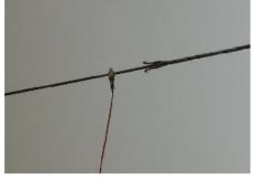
Conductor Grounding Clamp
