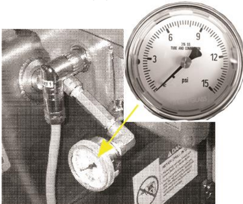
Figure B3. Replacement SF6 Gauge. Used on some Vista switches to replace defective internal gauges. Mounted on the SF6 fill port.
