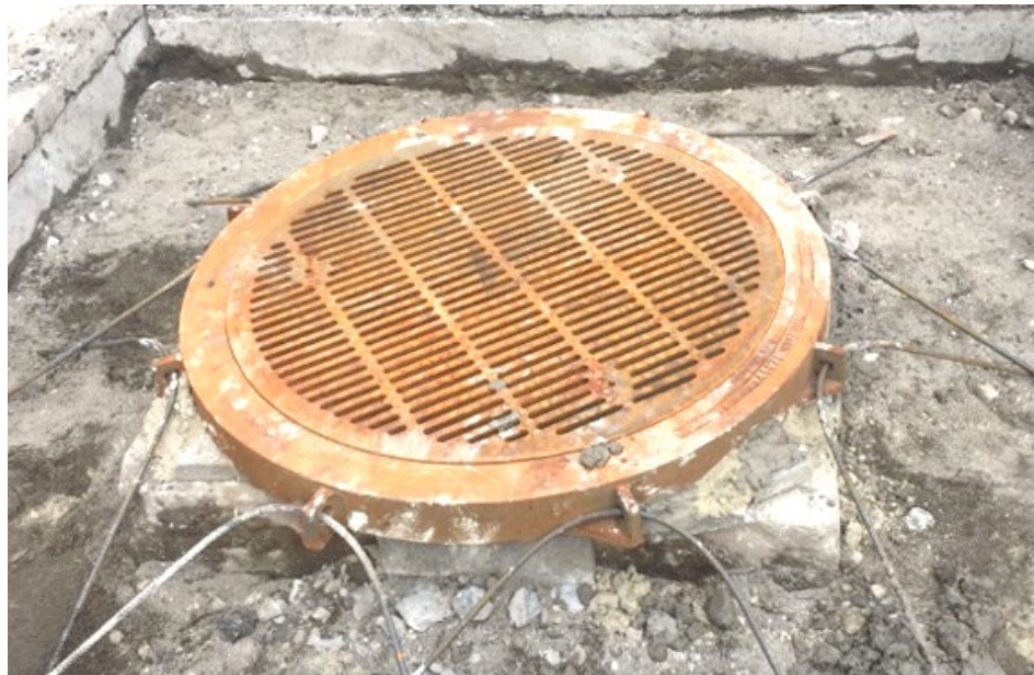
Figure 3a. Rebar Hairpin Example
