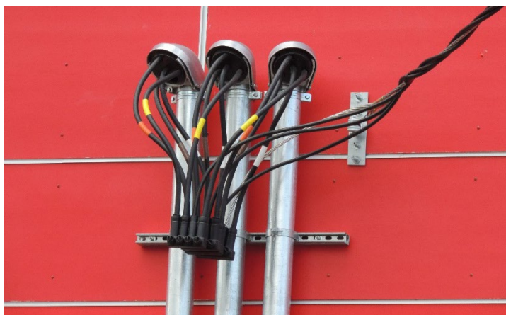
Figure 3.2b. Multi-Tap Insulated Connector, Stock. Nos. 013661 or 013662
