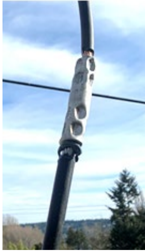
Figure 3.2c. Splice, Straight Compression, Staggered, Non-Tension, Secondary
