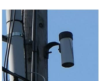
Figure 4.12g. Spare low-voltage fuse storage container (obsolete), SCL
