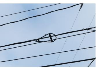
Figure 4.8f. Fiber optic cable storage bracket (a.k.a. slack halo or snowshoe)
