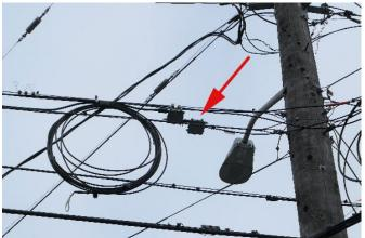
Figure 4.9f. CATV cable coupler (non-active), Comcast
