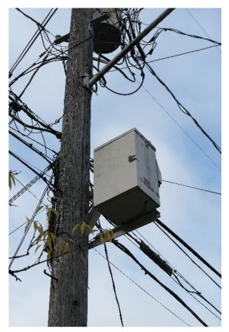
Figure 4.1q. Power supply enclosure, no SWF on pole, location of service disconnect switch
