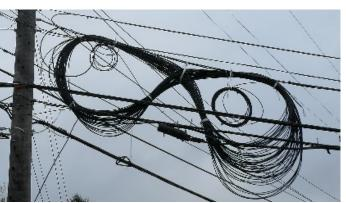
Figure 4.8k. Fiber optic cable slack loop (aka Figure 8 storage) waiting to be put in halo
