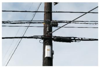
Figure 4.8c. Serving terminal (silver box) and splice case (center right) for telephone copper aerial cable
