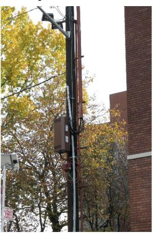
Figure 4.1I. Power supply enclosure and service disconnect switch
