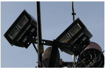
Figure 4.10c. Cluster-mount, LED floodlights; see SCL 1713.12
