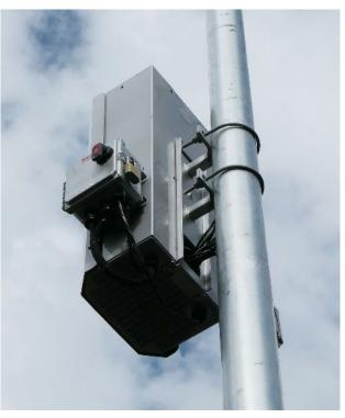
Figure 4.1v. SWF below streetlight bracket arm, co-located, enclosure
