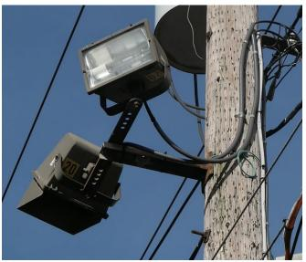
Figure 4.10b. Cluster-mount, high-pressure sodium (HPS) floodlights
