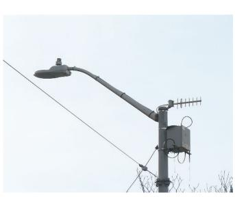
Figure 4.6d. ★ AMR microcell controller with Yagi antenna, PSE
