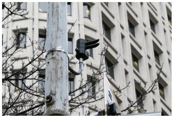
Figure 4.12e. Traffic signal pre-emption sensor
