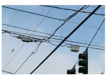
Figure 4.3a. Strand-mount antenna, Wi-Fi hotspot (at right)
