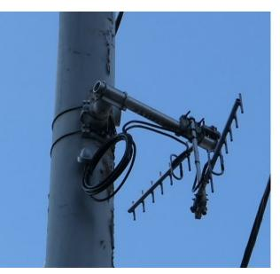
Figure 4.12i. ★Yagi antenna for King County Metro Transit
