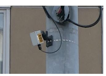
Figure 4.12b. SDOT device (Intelligent Traffic System (ITS) relay)
