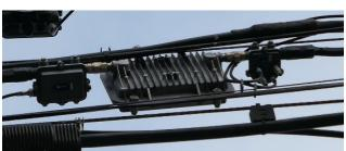
Figure 4.9b. CATV line amplifier, with coupler, WaveCom
