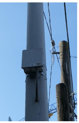
Figure 4.12j. Communications enclosure for King County Metro Transit Yagi antenna
