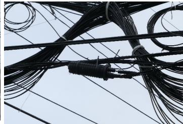
Figure 4.8I. Fiber Optic Cable Splice
