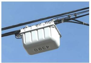
Figure 4.3c. ★ Strand-mount antenna, Wi-Fi hotspot, Comcast, alternate view
