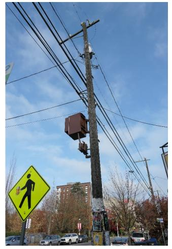
Figure 4.1p. Power supply enclosure, no SWF on pole, location of service disconnect switch, Crown Castle
