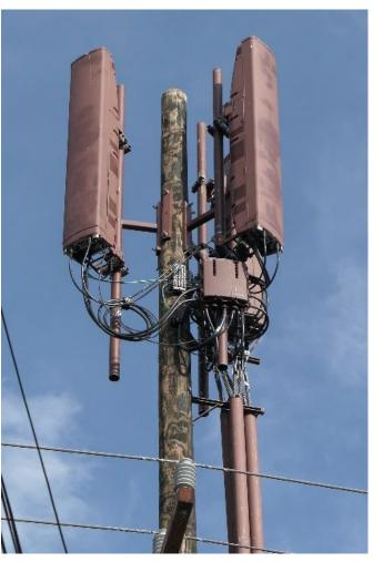
Figure 4.4d. **★** Macrocell antenna, T-Mobile
