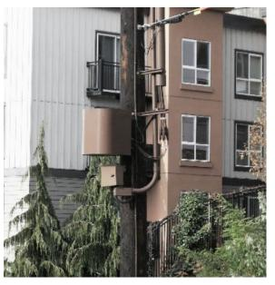
Figure 4.1i. Power supply enclosure and service disconnect switch
