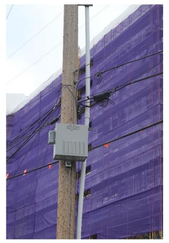
Figure 4.1r. Power supply enclosure and service disconnect switch
