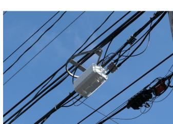
Figure 4.9d. Node amplifier, Comcast
