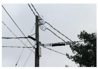
Figure 4.8b. Serving terminal (silver box) and splice case (center right) for telephone copper aerial cable
