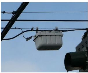
Figure 4.3b. ★ Strand-mount antenna, Wi-Fi hotspot, Comcast
