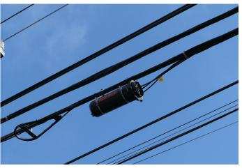
Figure 4.8h. Fiber optic cable splice
