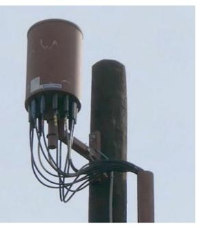
Figure 4.1k. ★SWF antenna
