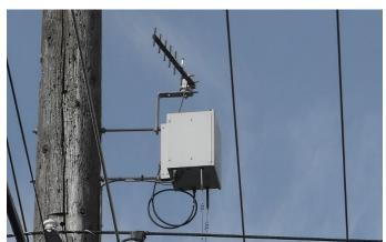
Figure 4.6f. ★AMR microcell controller with Yagi antenna, PSE
