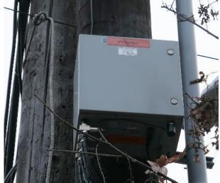
Figure 4.7c. Communications enclosure for AMI collector
