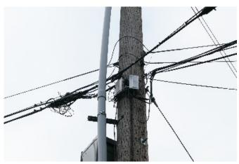
Figure 4.8d. Serving terminal for telephone copper aerial cable, alternate style
