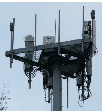
Figure 4.4b. ★Macrocell antenna on non-SCL monopole
