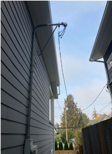
Figure 3.7.1.1g. Horizontal Mast with a Stiff-Leg Set
