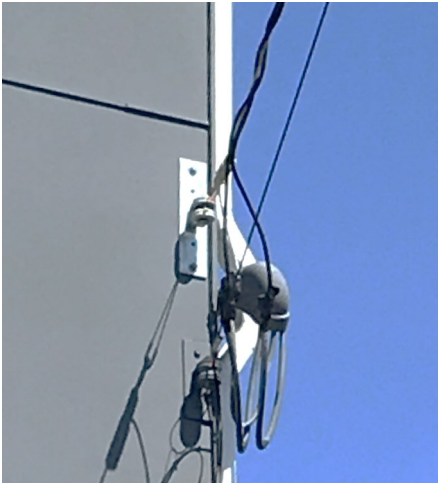
Figure 3.7.1.1g. Horizontal Mast with a Stiff-Leg Set
