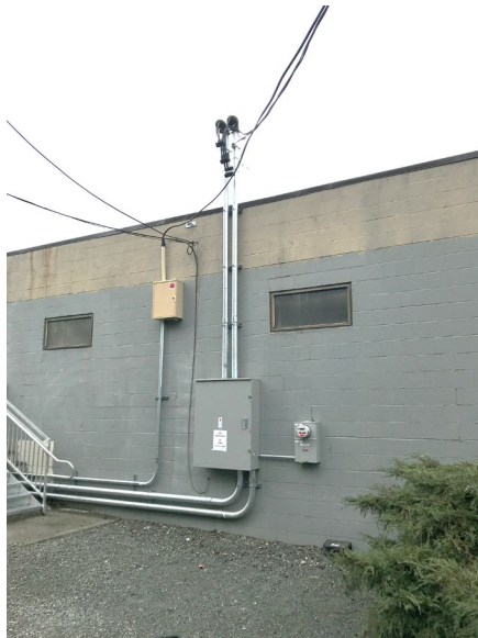
Figure 6.9.1. CT Service, Typical
