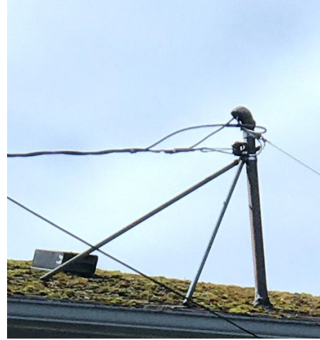
Figure 3.7.1.1f. Kindorf Bracket Attachment
