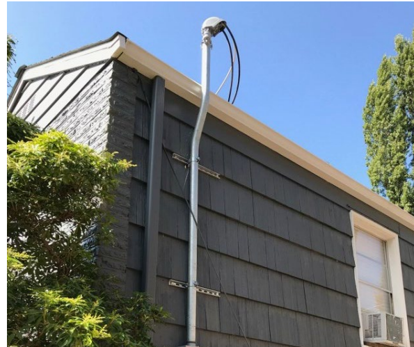
Figure 3.7.1.1h. Offset Bend without a Stiff-Leg Set or Back Guy
