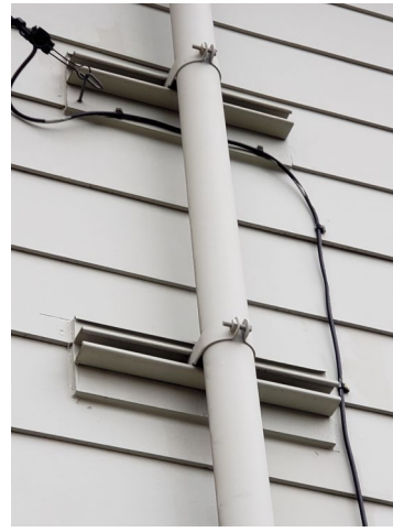
Figure 3.7.1.1h. Offset Bend without a Stiff-Leg Set or Back Guy
