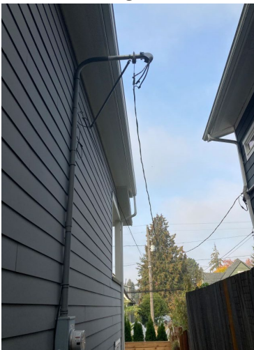
Figure 3.7.1.1g. Horizontal Mast with a Stiff-Leg Set
