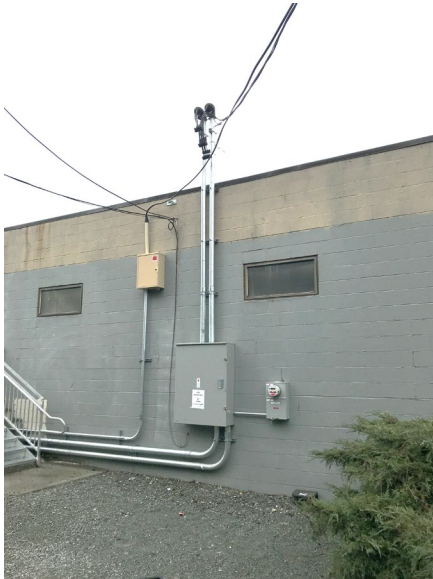
Figure 6.9.1. CT Service, Typical
