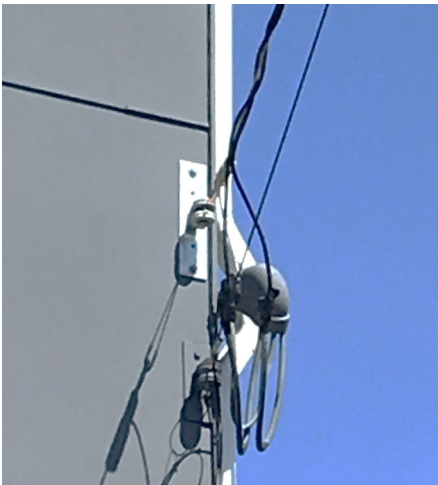
Figure 3.7.1.1g. Horizontal Mast with a Stiff-Leg Set
