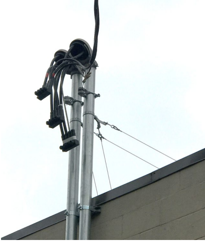
Figure 3.7.1.1.e. Service Bracket
