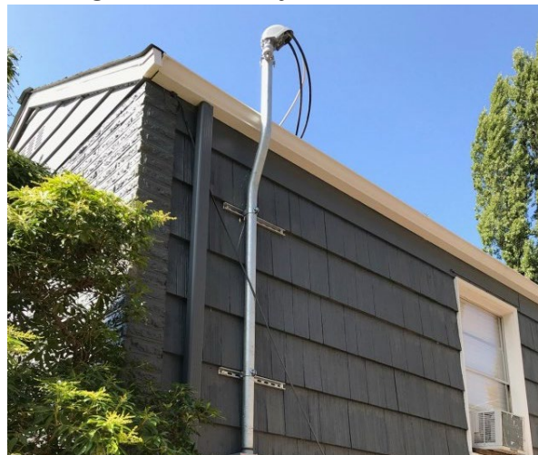
Figure 3.7.1.1h. Offset Bend without a Stiff-Leg Set or Back Guy
