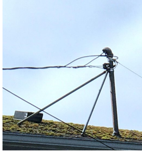
Figure 3.7.1.1f. Kindorf Bracket Attachment
