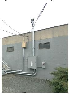
All transformer-rated meter sockets must have test switch provisions.
