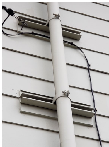
Figure 3.7.1.1f. Kindorf Bracket Attachment
