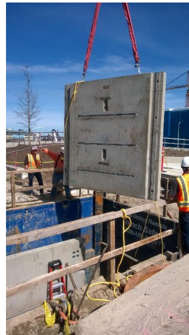
Figure 2. Precast Panel Vault
