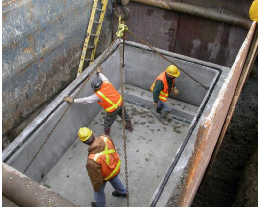
Figure 1. Precast Ring Vault
