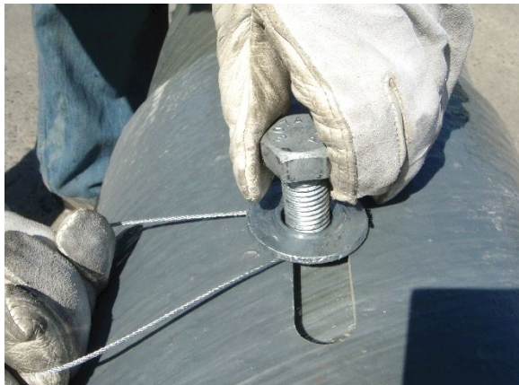
Figure 4b. Pole Module Joining Hardware
