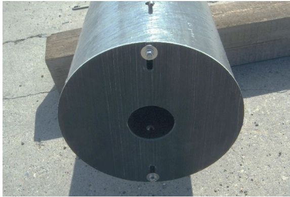
Figure 4d. Base Plate Fastening Hardware
