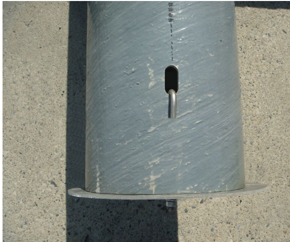
Figure 4e. Bracket Holes, 30-ft and 40-ft Poles
