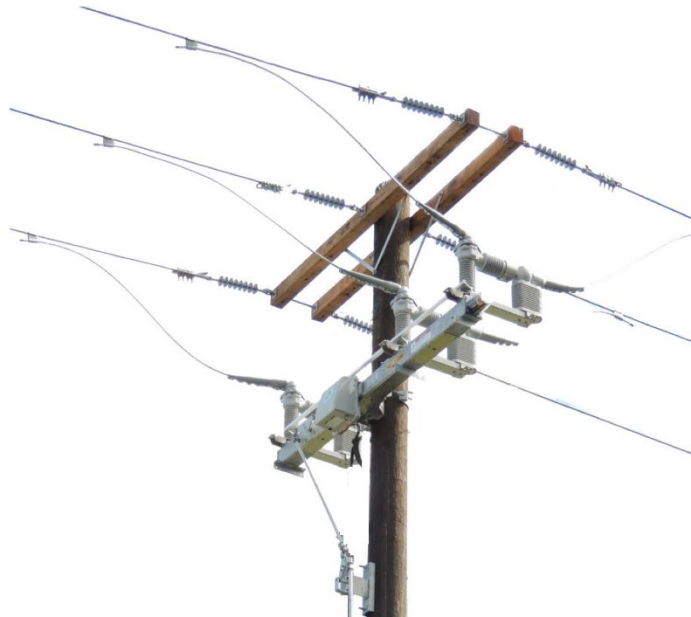
Figure 4.2a. Load Interrupter Switch, Horizontal
