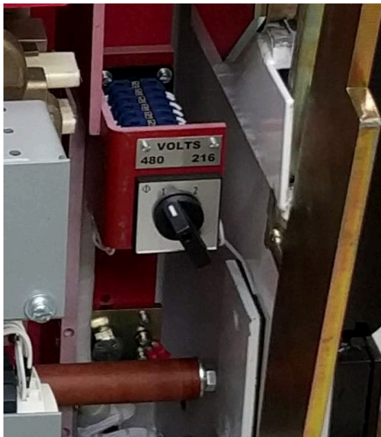
Figure 5.6. Voltage Selection Switch
