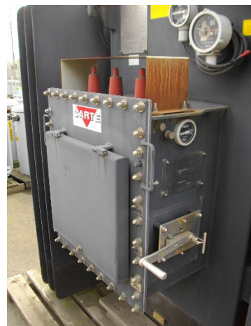
Figure 7.1, Bushing and Switch Chamber
