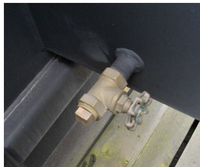
Figure 8.11f, Drain valve
