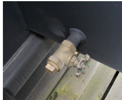
Figure 8.11f, Drain valve
