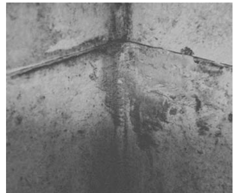
Figure 2. Mortar Patch for Spall Repair
