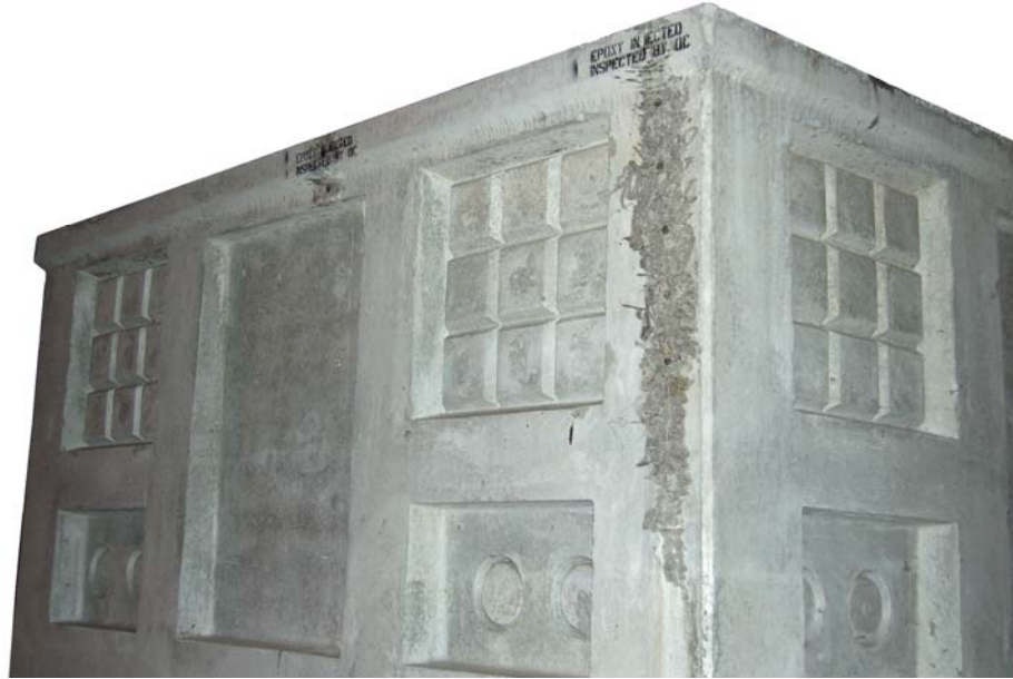
Figure 1. Vault Repaired with Epoxy Injection
