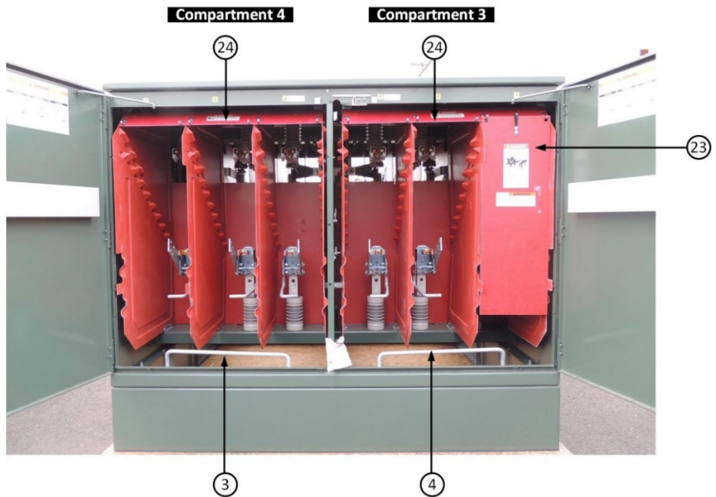
Figure 5c. PMH-9 Switchgear Compartments 3 and 4 Overall View
