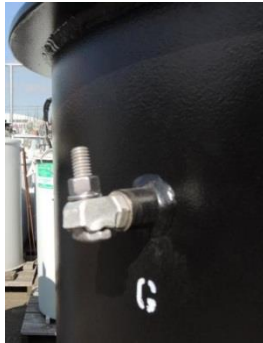
Figure 6.12.3a. Single-Phase Ground Lug
