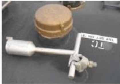
Figure 6.4. Tap Changer Access and Wrench
