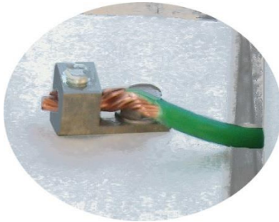
Figure 6b. Pole Ground Grounding
