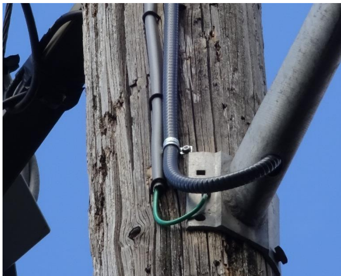
Figure 6c. System Neutral Grounding
