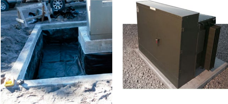
Figure 8b. Basic Concepts Geomembrane/Barrier Boom or SorbWeb Plus Blankets
