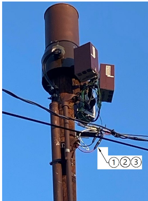
Figure 4b. Fusing Assembly (insulating boot, fuse holder, and fuse)
