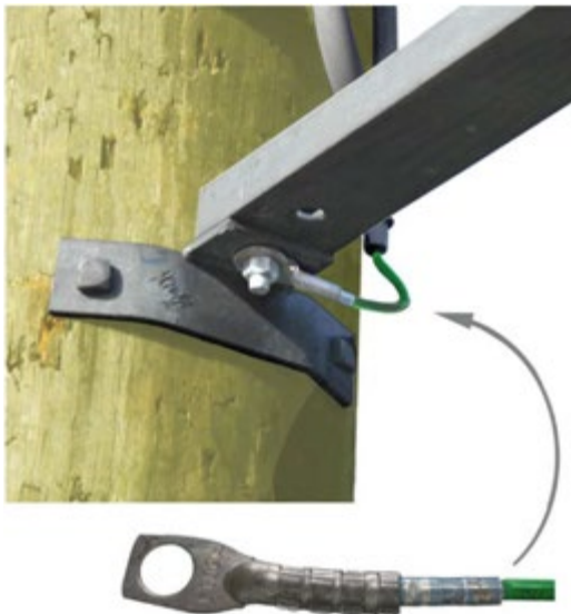
Figure 4c. Routing Ground Wire
