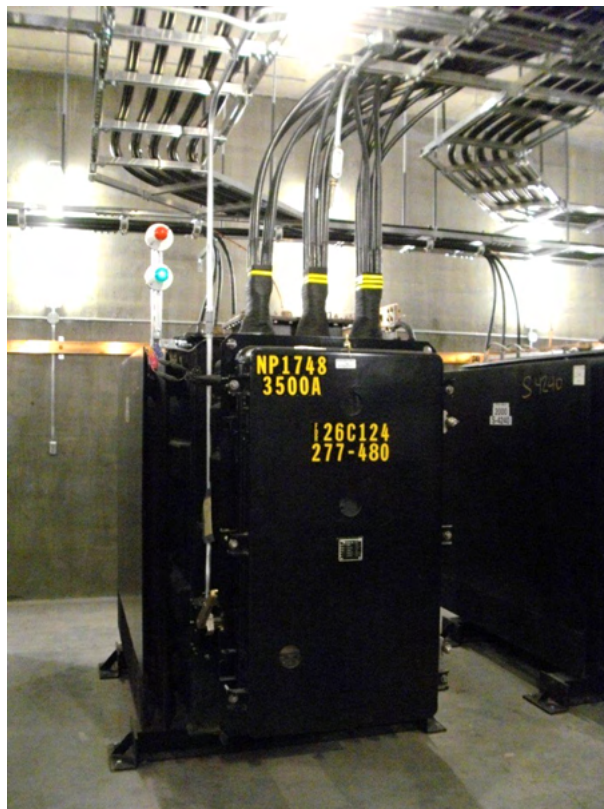
Figure 3.6a. Network Transformer
