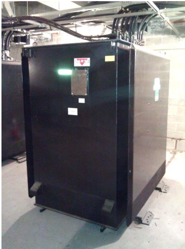
Figure 3.7a. Looped Radial Three-Phase Transformer
