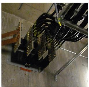
Figure 3.10e. Bus Bars Perpendicular to Floor, Plan View
