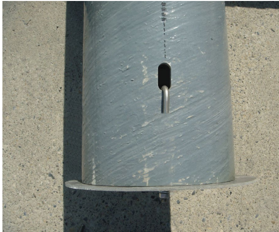
Figure 4e. Bracket Holes, 30-ft and 40-ft Poles
