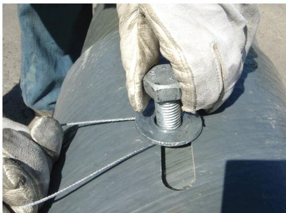
Figure 4b. Pole Module Joining Hardware
